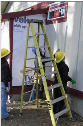
Thursday crew members work on siding
